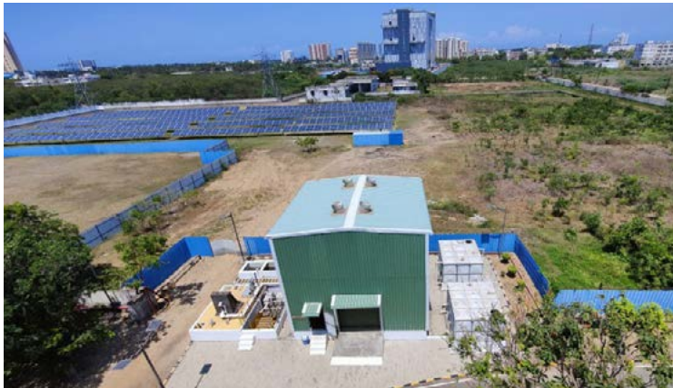
Advanced Sewage Treatment Plant, Chennai SIPCOT Campus, India
